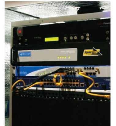
pCom® standard equipped with VSAT based IP voice, data switching, and LAN management.
